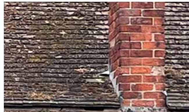
Limestone roof tiles
